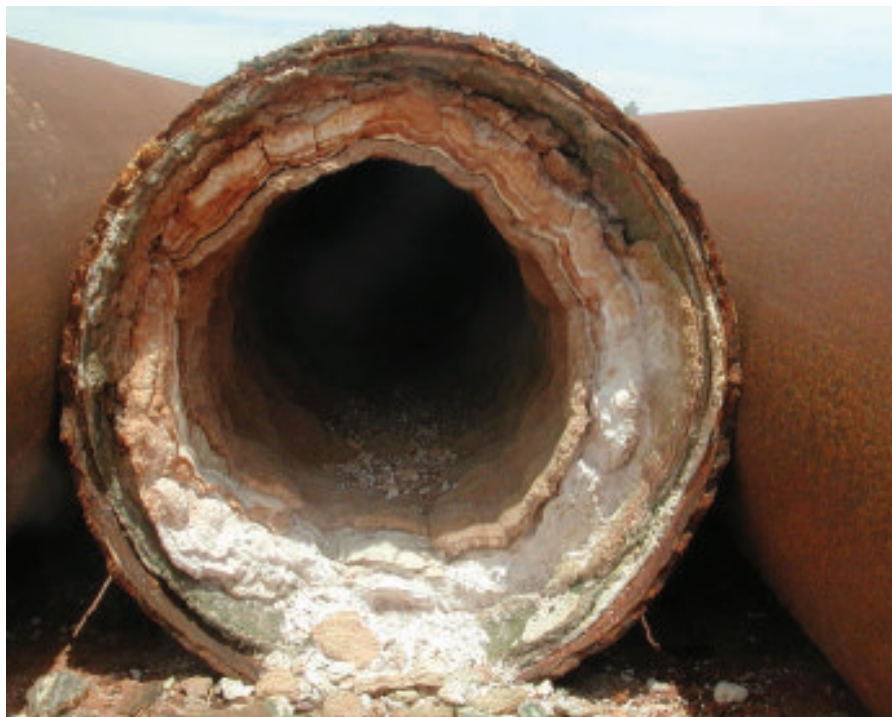
When water is heated, limescale can occur. This problem can clog pipes, reduce energy efficiency, and cause equipment failure. Courtesy: Scalewather North America Inc.
